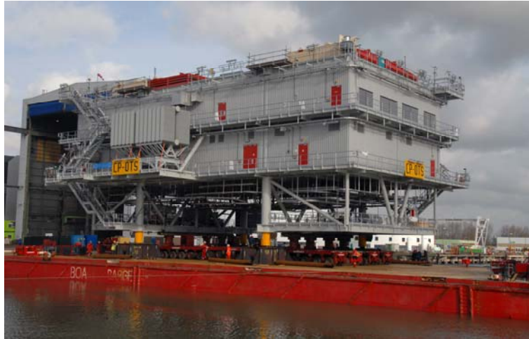
Load out offshore transformerstation
